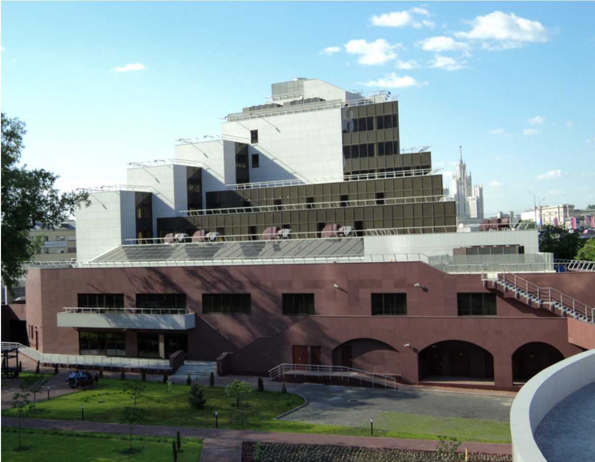
MKH-5 Project Moscow – ENKA Construction
