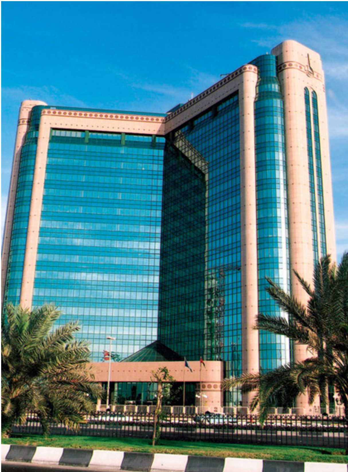
ATCO (ADNOC)- Head Office Abu Dhabi – Laing O'Rourke
