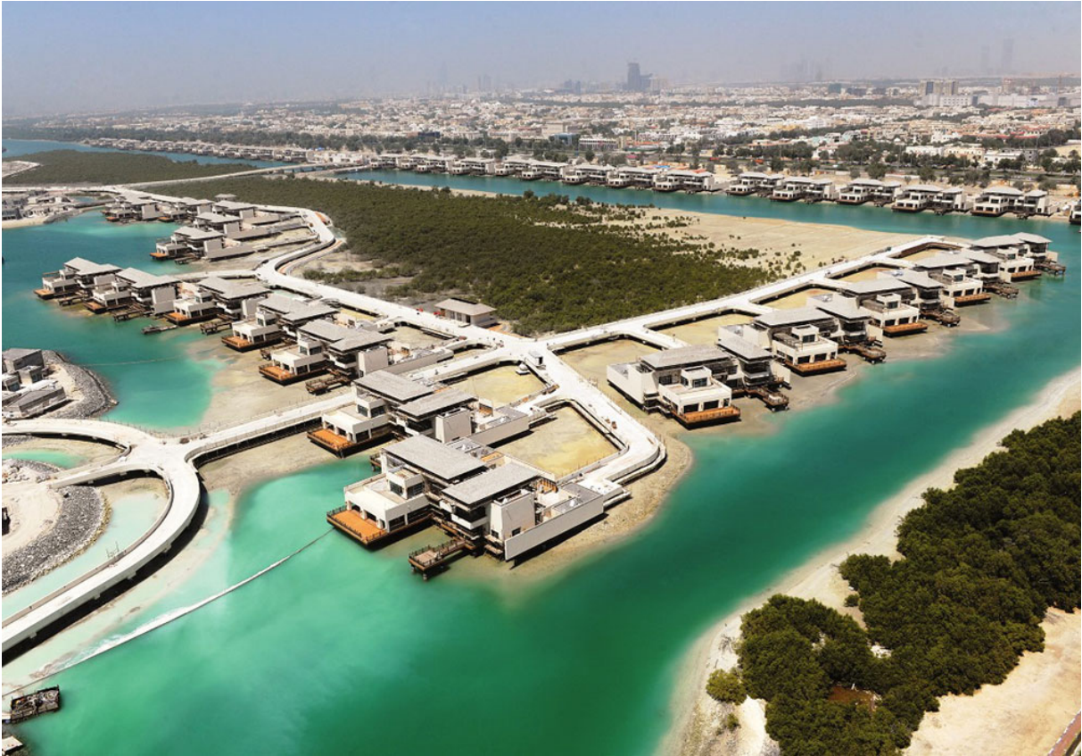
Al Gurm Resort Development – BESIX Abu Dhabi
