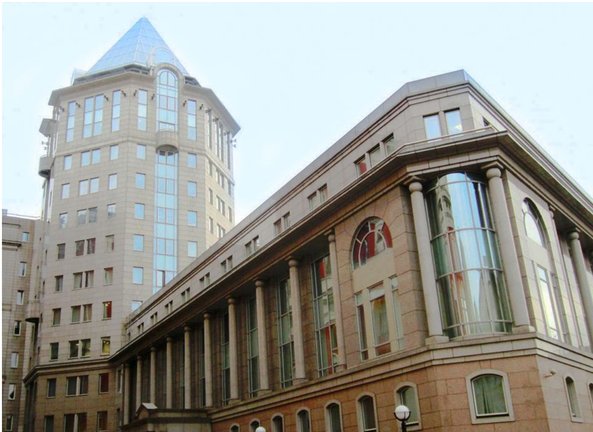
OFFICE AND SHOPPING BUILDING -USADBA CENTER MOSCOW
